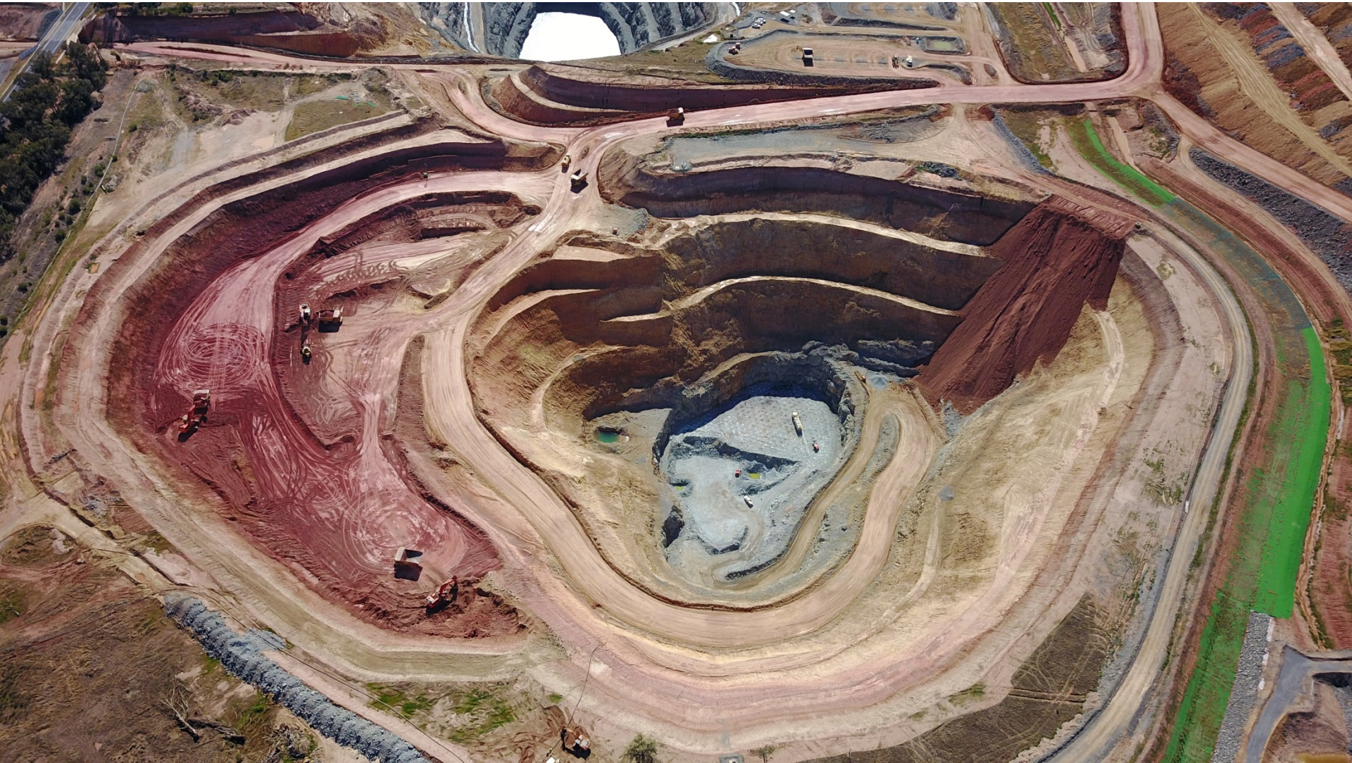
Current Caloma Two pit looking north
