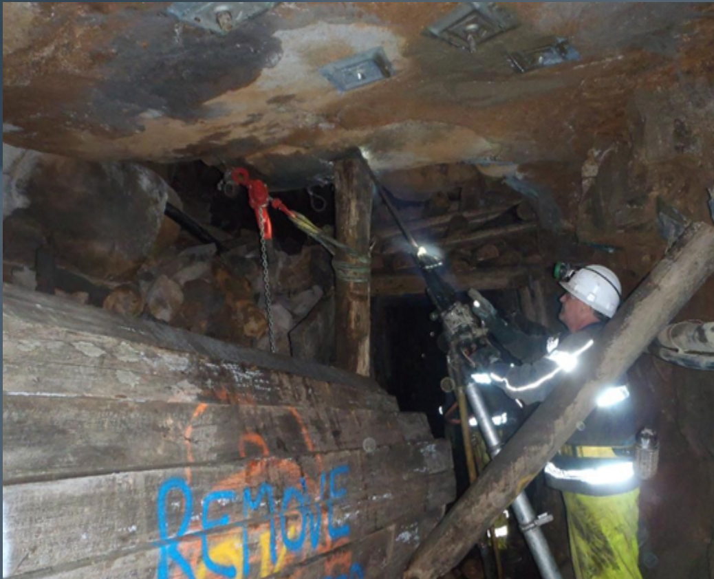
Above: Morning Star adit has been rehabilitated to allow diamond drilling to occur. May 2017
