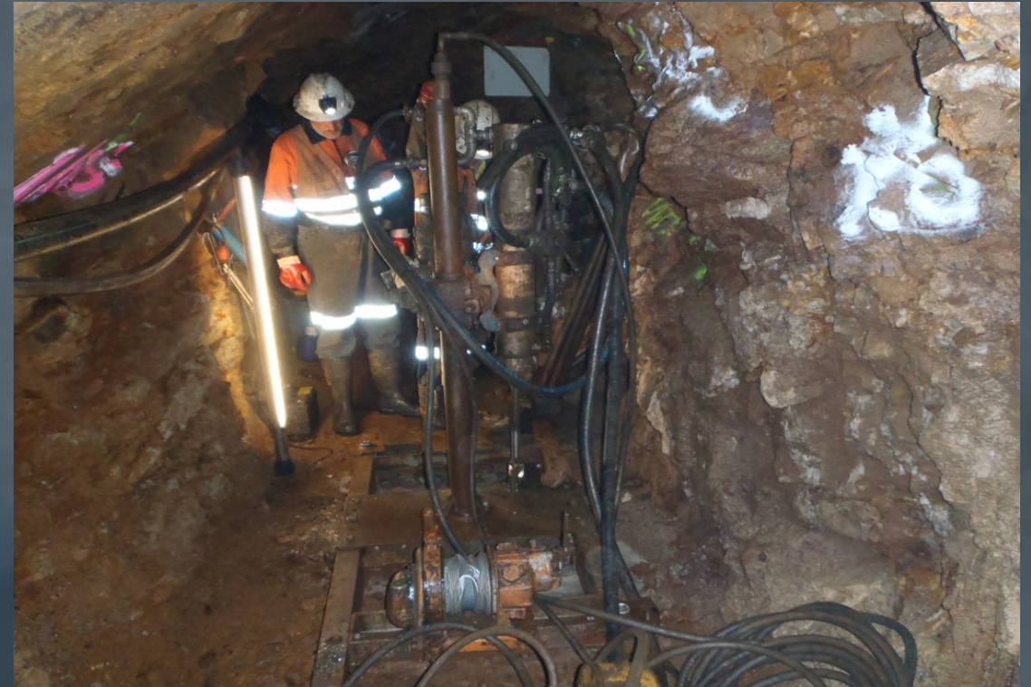
Below: Diamond drill in morning star adit, drilling the Stacpoole zone. June 2017
