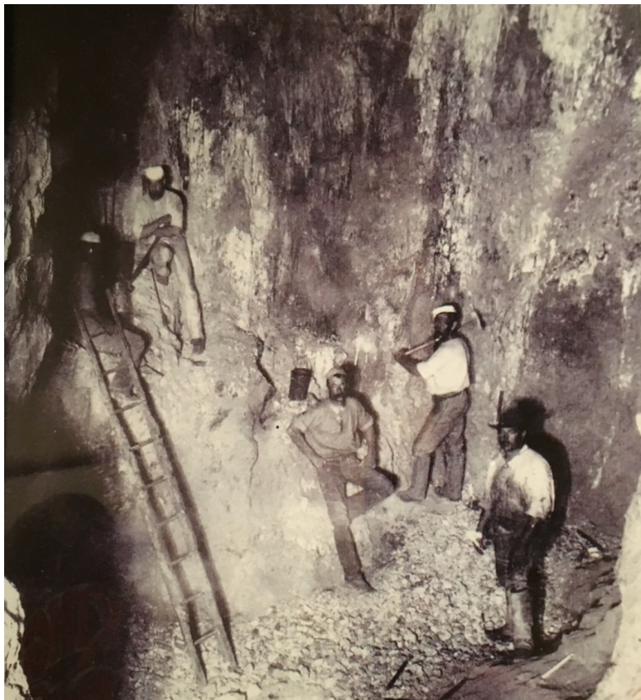
Stoping at the Nymagee Copper Mine (Date Unknown)
